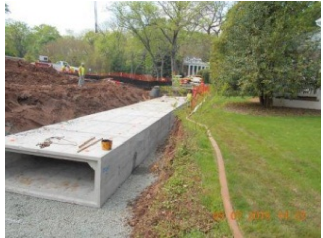
Upper Flat Branch Interceptor Project
