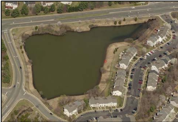
Cockrell Branch Stormwater Pond
